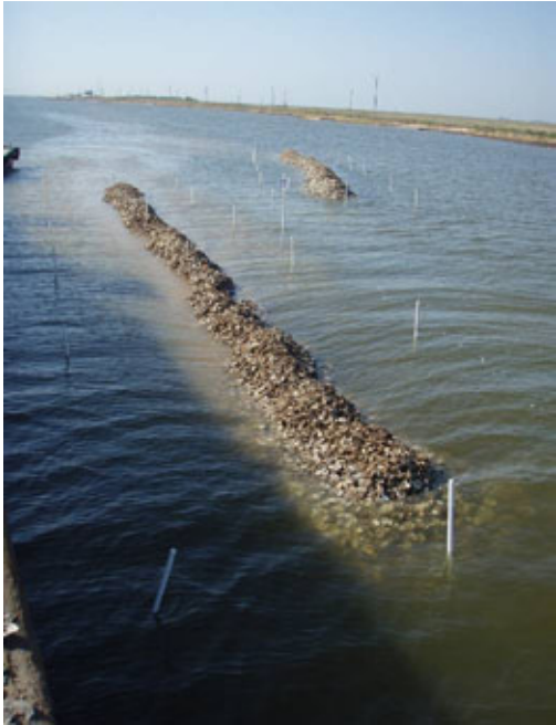
Completed Reef at Alabama Port
