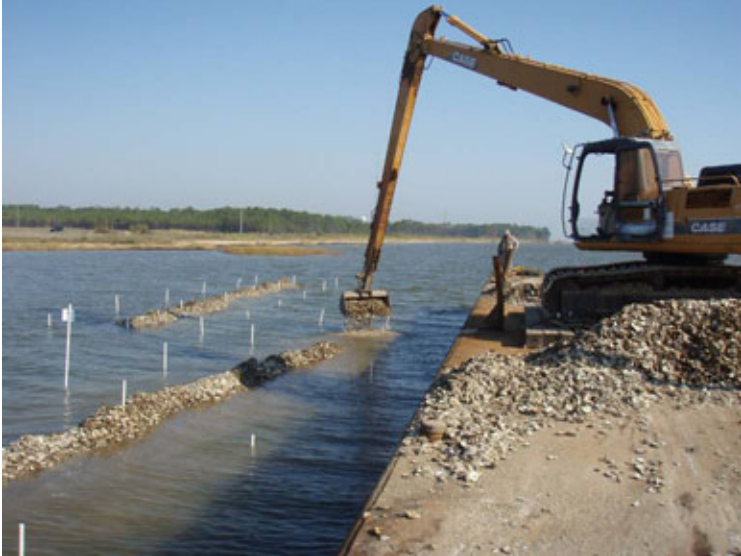
Reef Construction at Alabama Port
