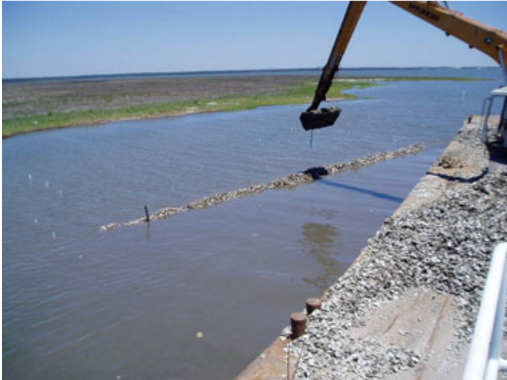
Reef Construction at Point aux Pines
